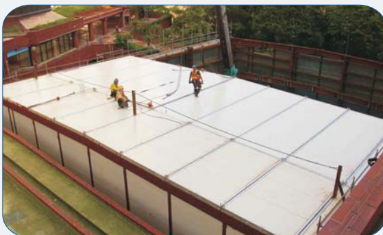
Lei Tung Estate - MTRC Project
